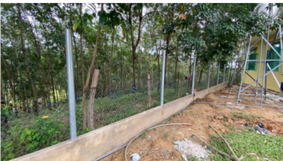
The new safety fence was built up
