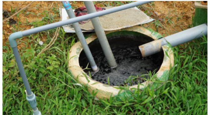
The storage tank for liquid compost
