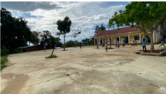
The new playground was built
