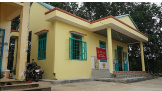
The front of New School with new painting and new roof
