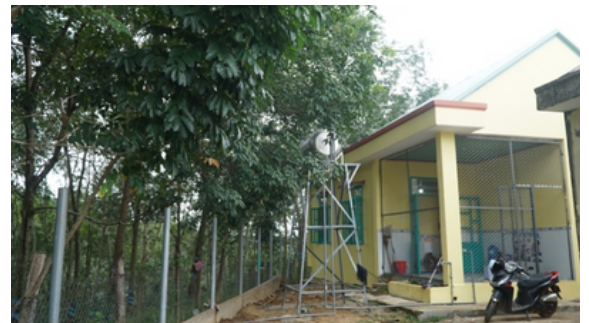
New inox water tank was installed
